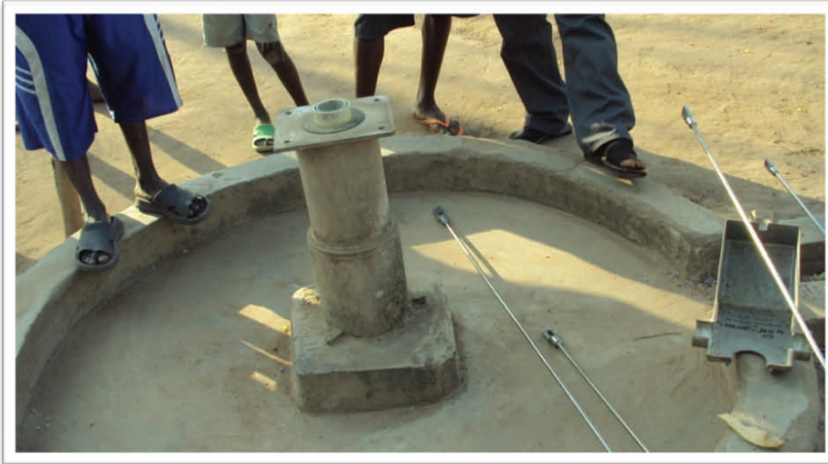
The previous water source
