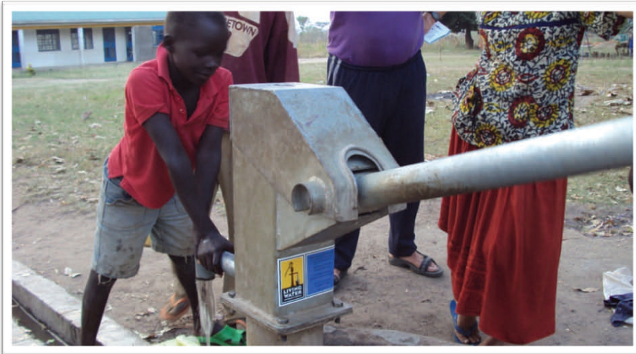
Close-up of the new water pump and plaque
