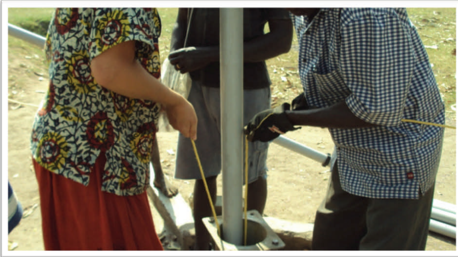
Project in process
