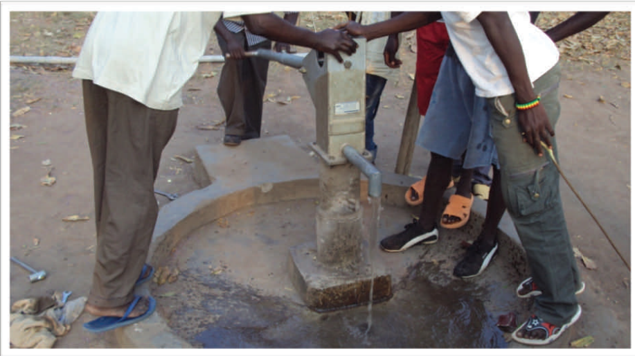
Pumping the first stream of clean water
