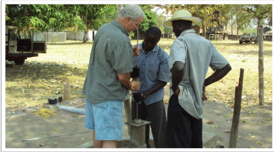
Project in process
