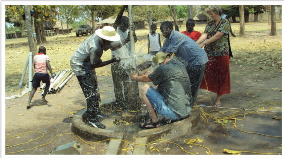
Project in Process
