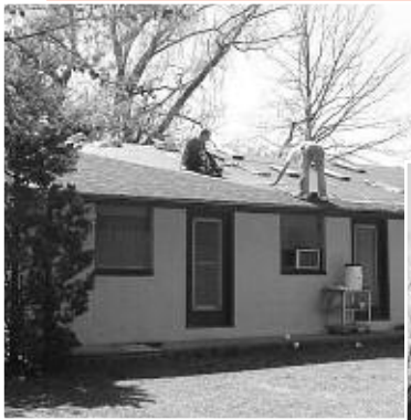
Removing old shingles
