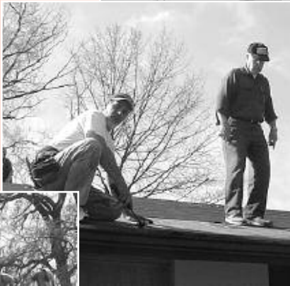
Removing old shingles
