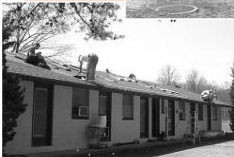
Surveying the progress
