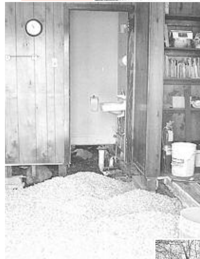
Spreading stone - preparing for concrete floor
