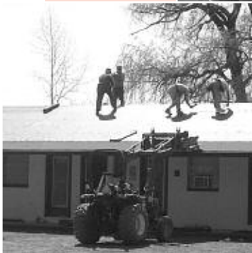
Using front end loader to hoist new shingles onto roof
