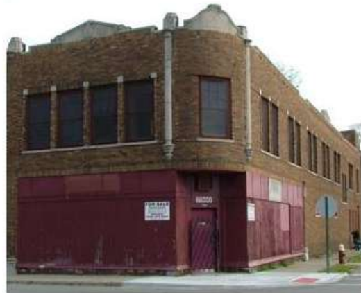
Above: New Mack Building
