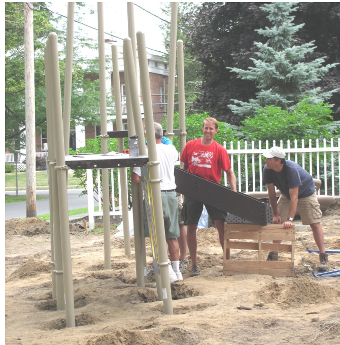
Pastor Dirk Gieser, Tom Orsini and Scott Carlton, starting playground construction, 2011.
