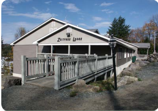
Exterior of building
