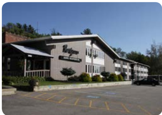
Exterior of building
